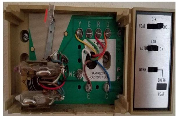
Option 2: 2 Stage heating w/ emergency heat. Single wire (W2 or AUX)
